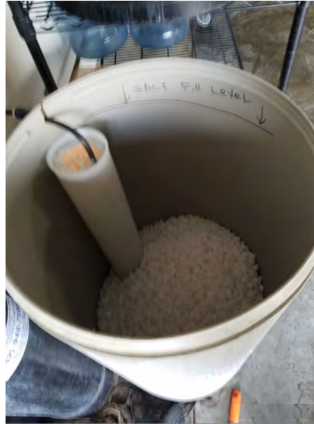
Water softener Brine tank salt level...
